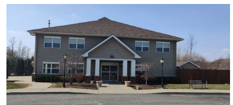
Nelson Hopkins Apartments
